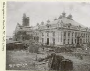
Building the sewage disposal plant on New Jersey Ave., SE, around 1906.
